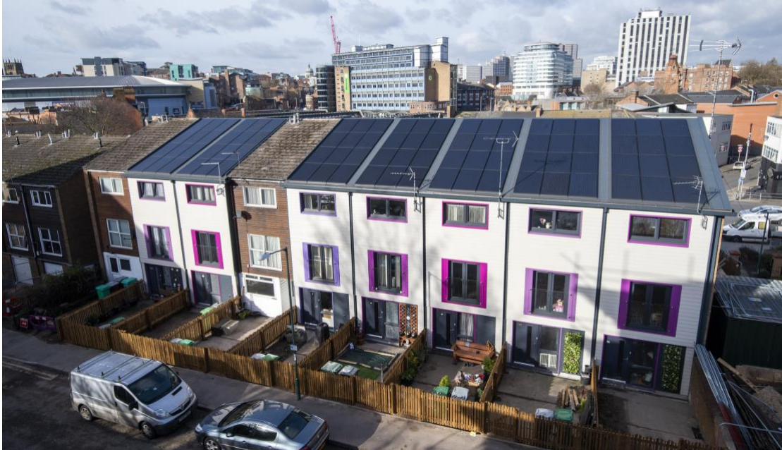
Nottingham – Energiesprong applied to 7 of 9 properties in a terrace.
